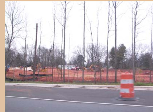
A new mixed-use development provides connectivity between downtown and NC-51. The project includes a natural buffer along the highway frontage.
