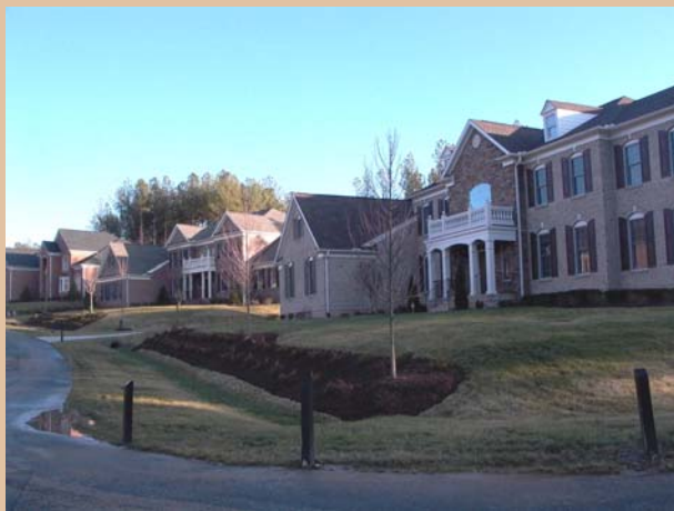
New clustered subdivisions in southwest Cary do not have curb, gutter and sidewalks, and instead use swales to manage stormwater runoff.
