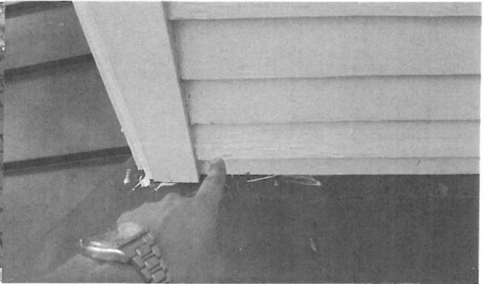
Upper front right, rotten siding
