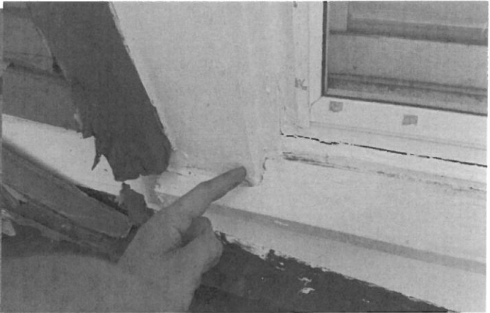
Upper right window, left trim board rotten.
