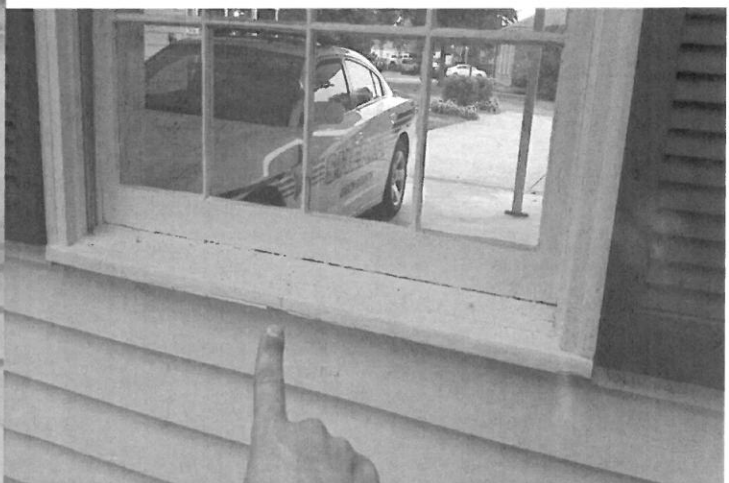
Back of the carport rotten window sill nosing
