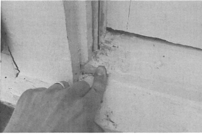
Upper, front right of bay window, rotten window sill.
