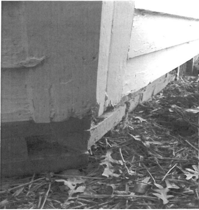
Front left of bay window, wood is solid, but Would recommend sealing the bottom edge.
