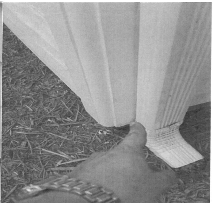
Lower right back corner board rotten
