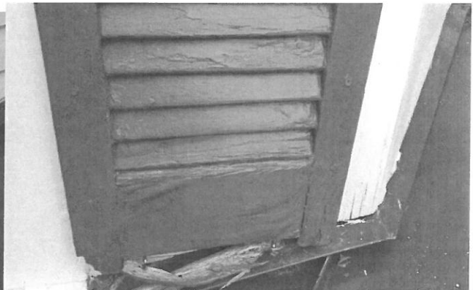
Above patio, right of bay window, shutter is rotten, can only Repair the rotten wood by piecing in new wood.
