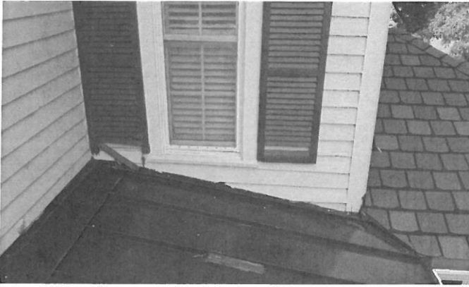
Upper front right, repair damaged shutter. Because These are old and custom, we can only piece in new Wood, and make it match existing
