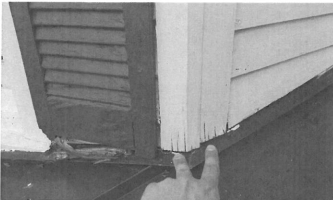
Above patio, right of bay window, both corner boards Are rotten.
