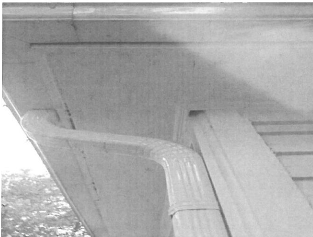
Cracks in the soffit back of the carport, needs caulking
