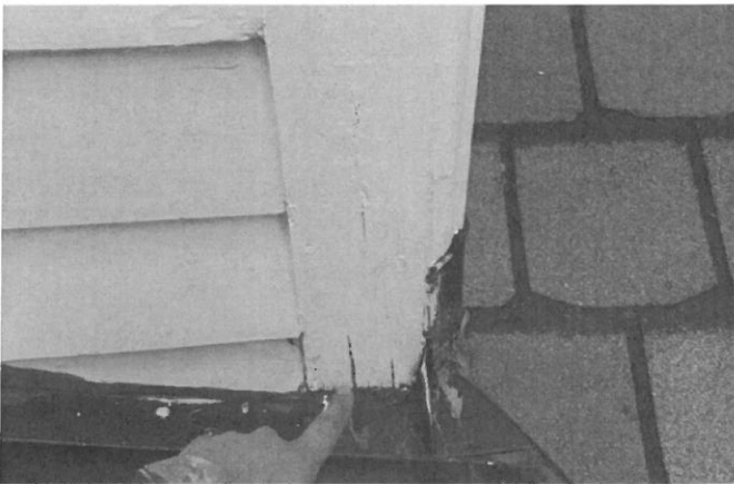
Upper right corner board, rotten.
