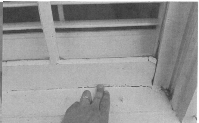
Upper windows above patio, rotten sash, can only repair Bad wood, no replace wood available.
