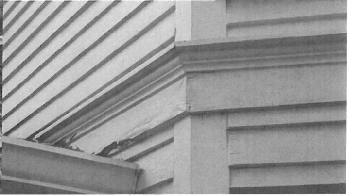
Front left of bay window, both bed moulds are rotten, and both Trim boards underneath are rotten.
