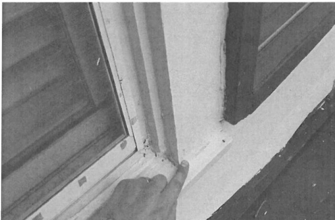
Upper right window, right trim board rotten.
