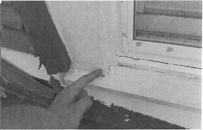
Upper right window, left trim board rotten.
