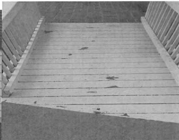
Front left ramp, peeling paint
