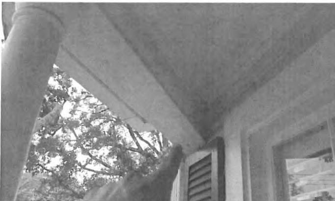
Front patio inside, left. Rotten back fascia and trim board.
