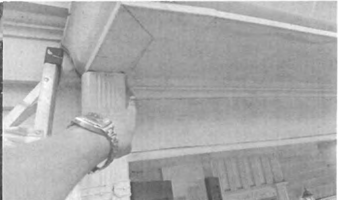
Front Patio, left side, rotten bed mould
