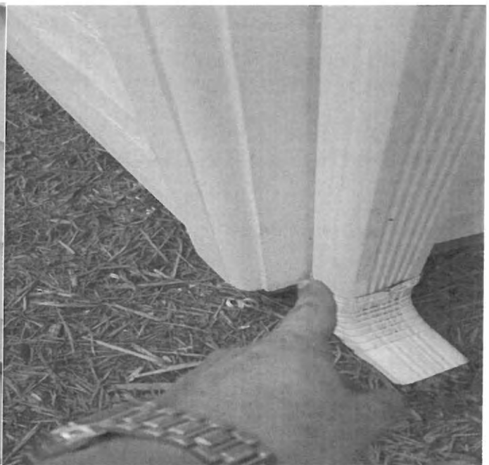
Lower right back corner board rotten
