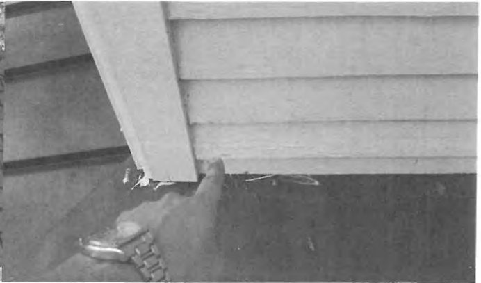
Upper front right, rotten siding
