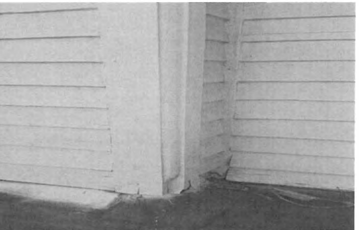
Upper left front, two rotten corner boards and quarter round And siding
