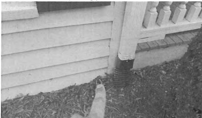
Front right of bay window, rotten siding
