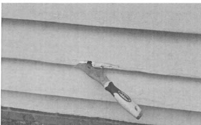
Right side of carport, rotten siding
