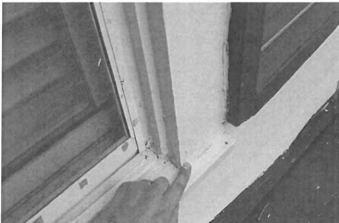
Upper right window, right trim board rotten.
