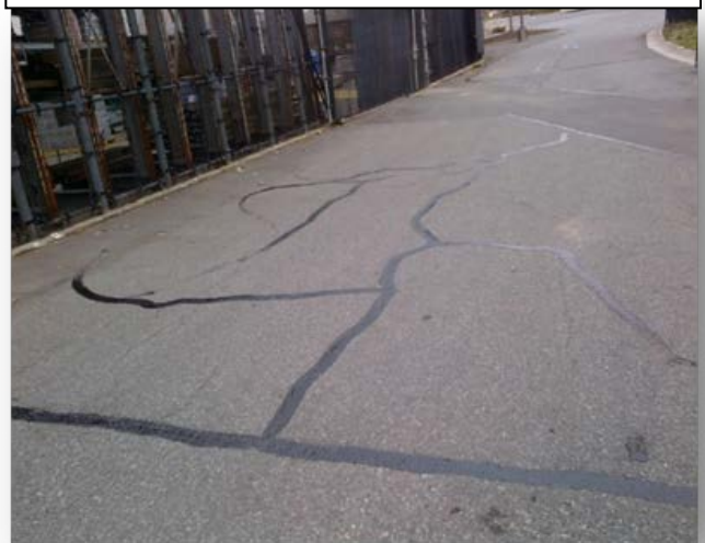
Lowes University area Charlotte NC (hot crack filling)
